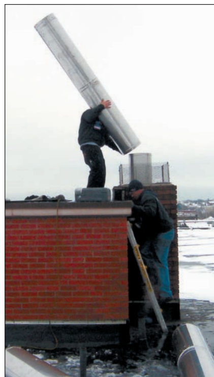
A rigid liner being assembled.
