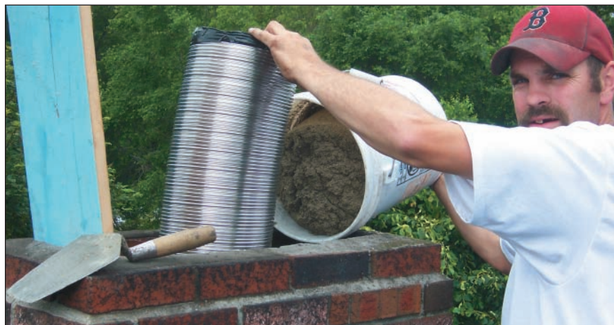
Installing mixed insulation around the liner.
