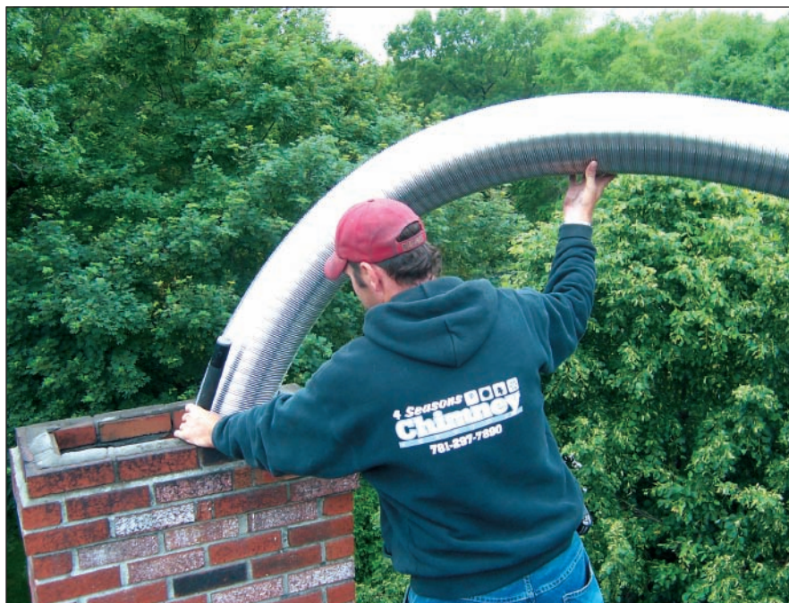
Flex liners are the most common type, and must be used for relining chimneys with offsets.
