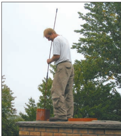
The chimney should be cleaned thoroughly before relining.
