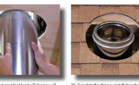
10. Complete the chimney installation above the roof by adding more chimney sections. Make sure the chimney is plumb.
