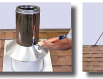
13. Slip storm collar around chimney and slide down. Apply high temperature silicone sealant where storm
