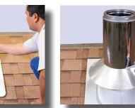
12. Add more chimney sections until chimney is at least 3 ft above roof, and at least 2 ft above any part of your collar will meet chimney
