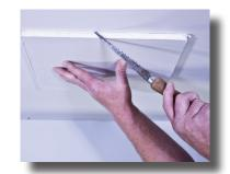
1. Drop a plumb line to center of stove flue collar. Mark center point on ceiling. Refer to installation instructions for framing dimensions.
