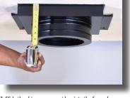
2. Slide the chimney support box into the framed opening from below, and level it. At least 2" of the box should extend below finished ceiling.
